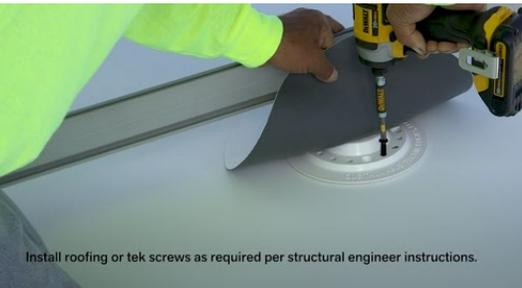
Install roofing or tek screws as required per structural engineer instructions.
