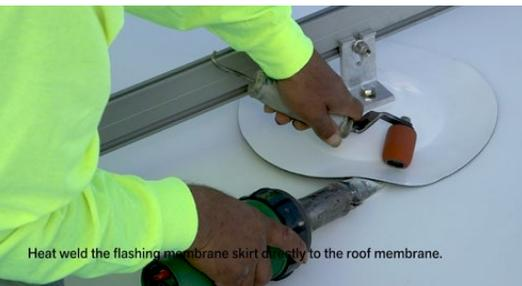
Heat weld the flashing membrane skirt directly to the roof membrane.
