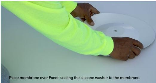
Place membrane over Facet, sealing the silicone washer to the membrane.
